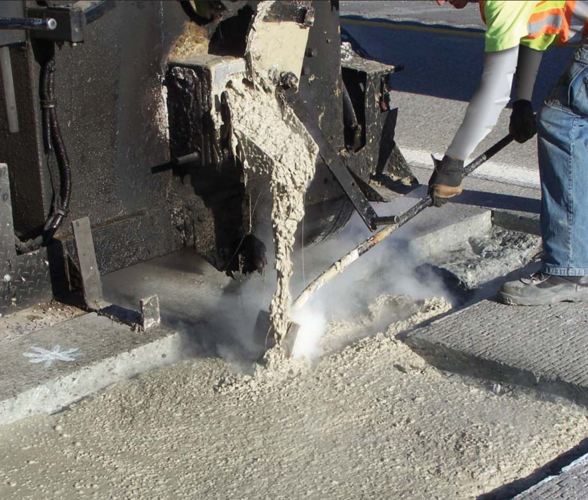
Four-corner, corner break repair
