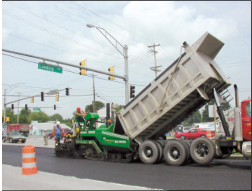
*The hot-mix asphalt industry chose two Superpave mixes to use in rebuilding its intersection, the corner of Route 40 and Maryland Route 213 near Elkton, Md.*
