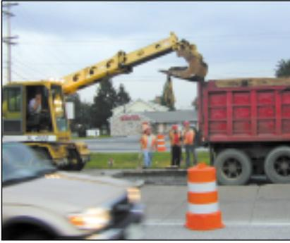
*Gradall excavators with stripping buckets were used for concrete removal.*
