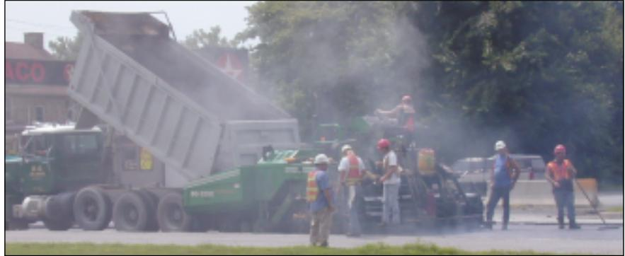
*The paving operation consisted of one Barber Greene 225 paver.*
