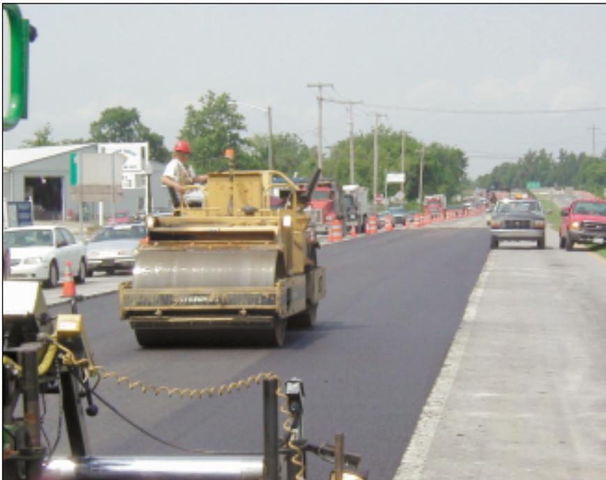
*Faced with a rutting problem, the Maryland State Highway Administration decided to compare the performances of hot-mix asphalt and portland cement concrete by giving each industry one intersection to rebuild along U.S. Route 40.*
