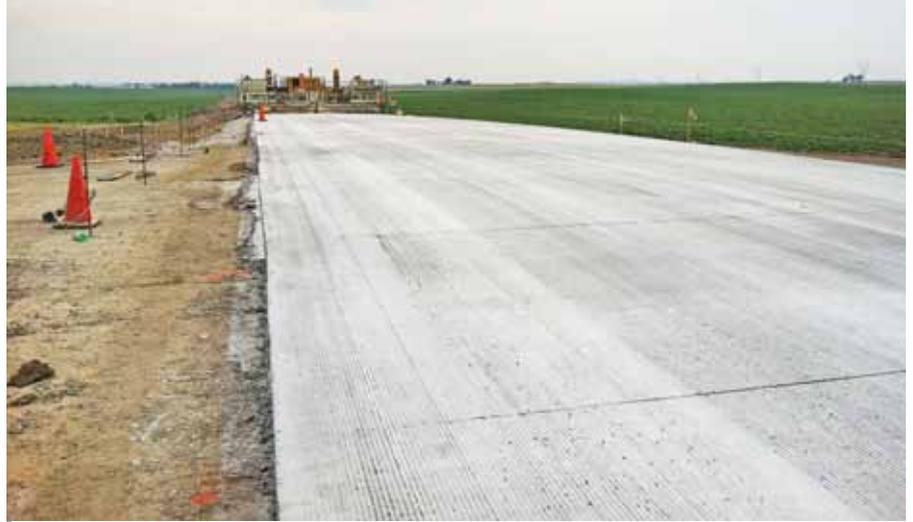
The flexibility of using PCC as a construction material has been much improved in Iowa through the use of the maturity method. Better admixtures also have allowed crews to transport mix over greater distances and with larger placement windows.
