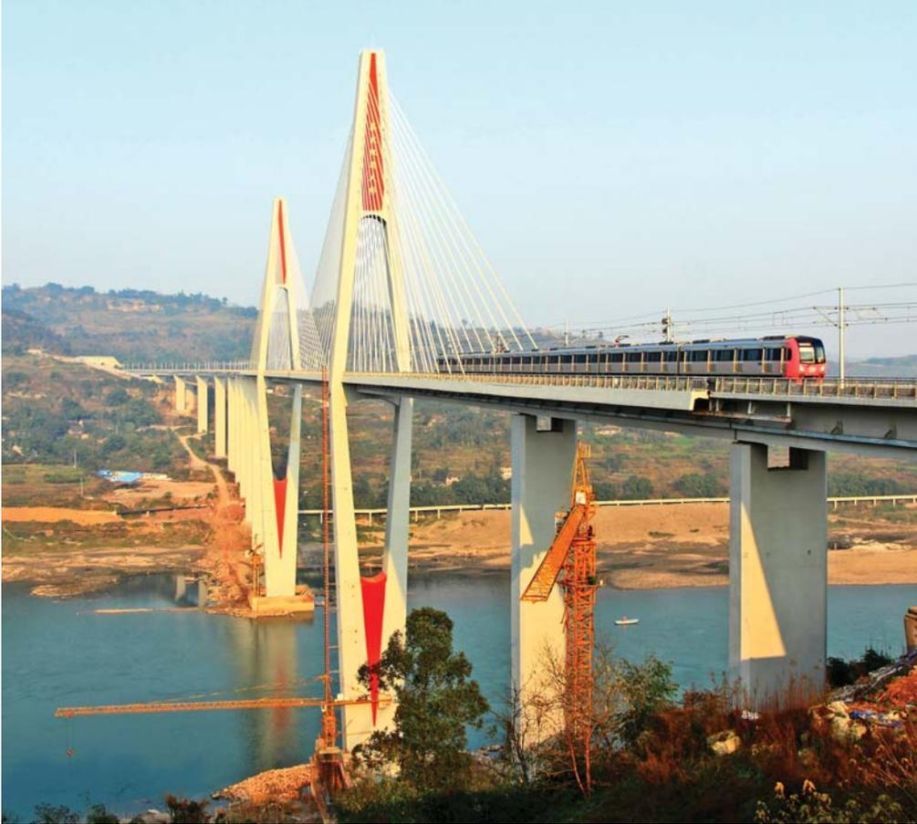
To compensate for the narrow appearance of the girder, a diamond-shaped tower was selected for the Caijia Bridge to provide a more solid, substantial appearance.
