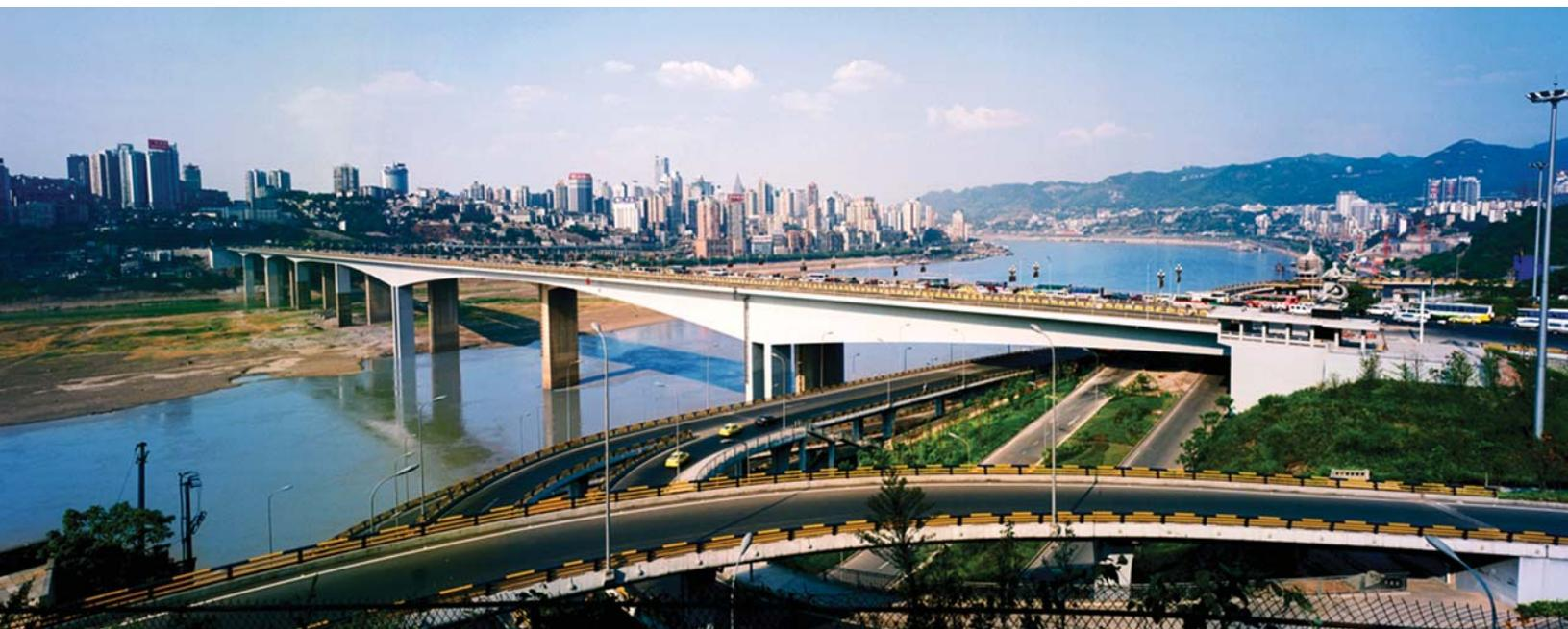
For aesthetic reasons, as well as to streamline water flow, the piers of the Shibampo Bridge were placed adjacent to the old bridge piers, necessitating the same span arrangement. After extensive study, the Chongqing Waterway Bureau decided that the pier between the existing main navigation channels must be removed. Consequently, the main span of the new bridge is about 1,083 ft.
