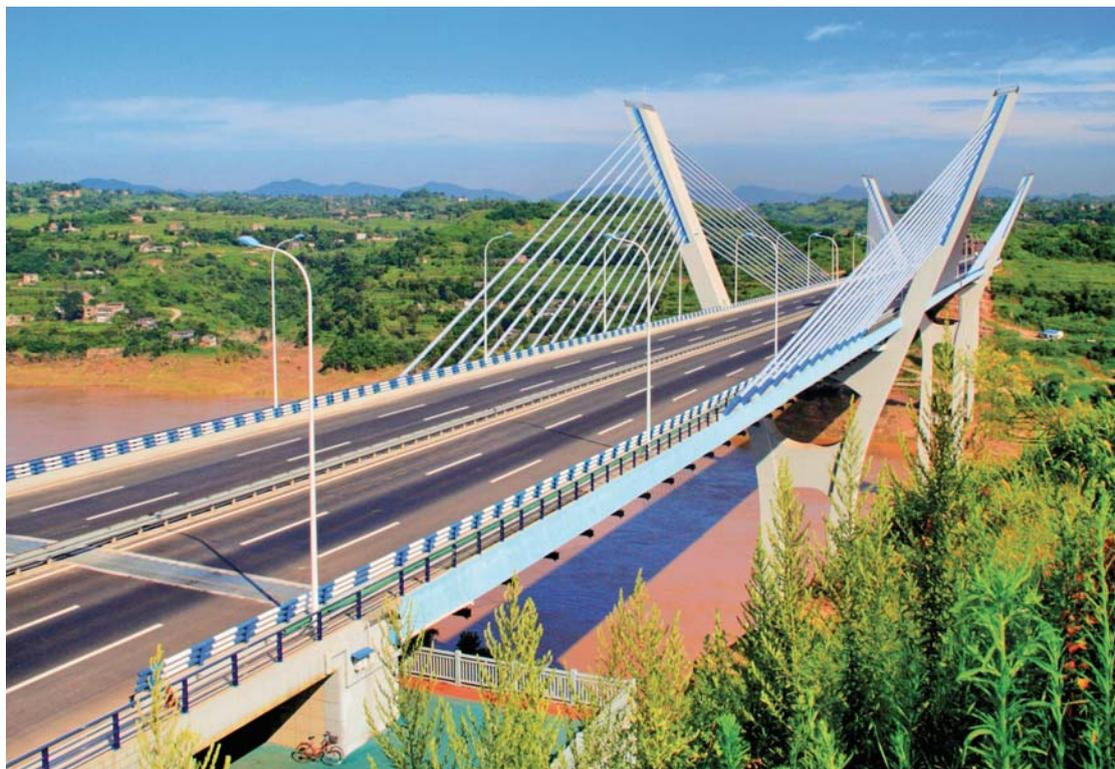
**Not only do the inclined tower columns of the Jiayue Bridge offer bridge users panoramic views, but they also create a widening effect that breaks up the monotonic appearance of the tall towers.**
