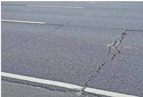
5. Existence of reflective crack patterns matching typical PCC joint patching geometry;
