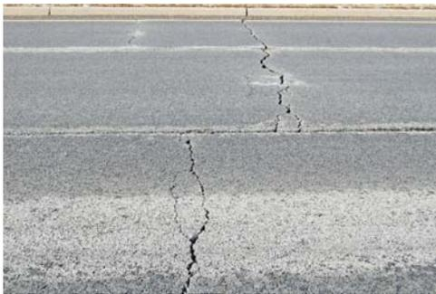
Figure 2. Existence of crack patterns resembling utility cuts in PCC pavement.
