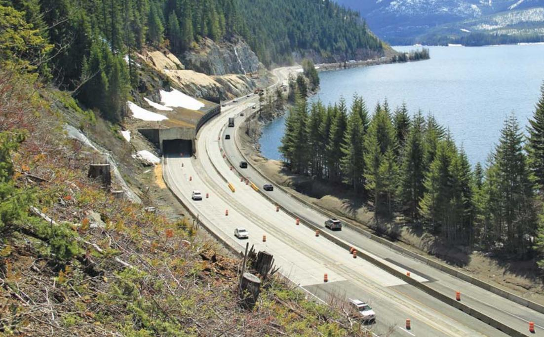
Atkinson Construction proposed a Cost Reduction Incentive Proposal by which an existing snowshed was to be removed and replaced with two new avalanche bridges.
